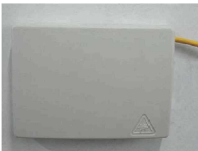
Pic22: cover the terminal box
