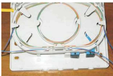
Pic14: after shrink, splice protective slot tube put into the slot of tray
