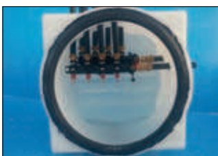
Ground source heat distributors
